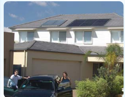
Grid Connected solar installation Sydney, Australia.
